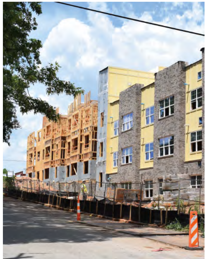
Image: senior housing development under construction in the Subarea Source: McAfee3
