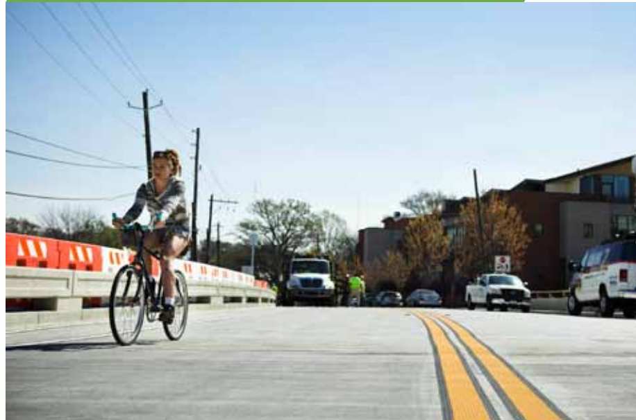
After one year of construction, the Edgewood Avenue bridge is now open. Photo credit: Christopher T. Martin.
