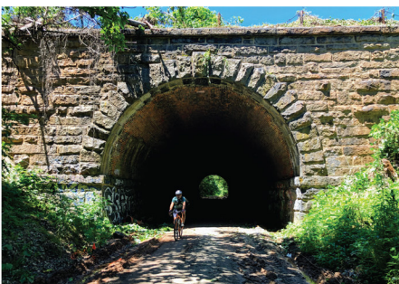
Above: Southside Interim Trail tunnel under Hank Aaron Dr./McDonough Blvd. Photo: John Becker.
