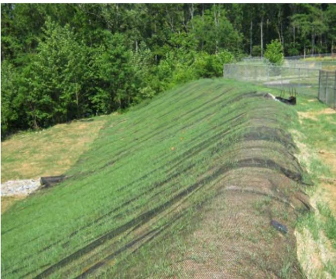
Typical erosion control and slope stabilization techniques.
