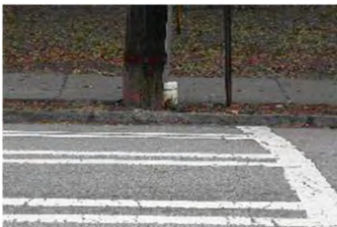
Figure 21 – Obstruction at Crossing at Cherokee Avenue and Glenwood Avenue
