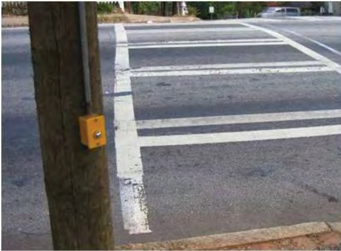
Figure 46 - Pedestrian Button with Inappropriate Placement
