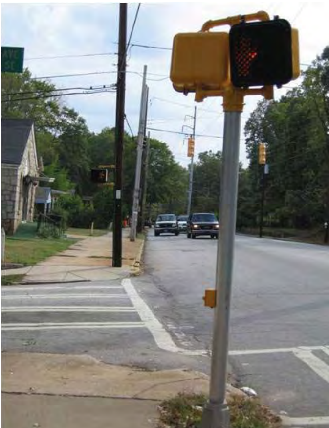
Figure 47 - Disoriented Pedestrian Signal Head
