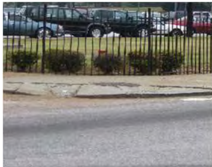
Figure 29 - Corner at McDonough Boulevard and Boulevard buffer zone. A considerable amount of obstructions (poles, posts, bushes and trees) limit the walkway passage to an insufficient width. Figure 30 and Figure 31 show some of the issues described.
