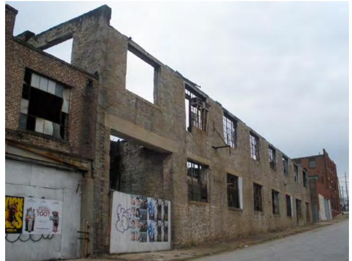
This historic building on Stephens Street is falling apart, but its walls could still be incorporate into new development
