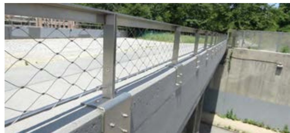
The existing bridge over North Avenue is adapted for the Atlanta BeltLine trail with safety railings
