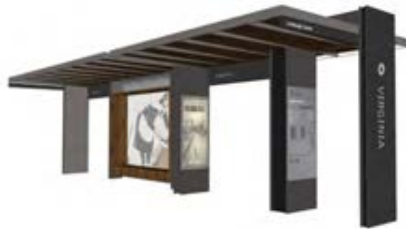
Transit Station Typology - The station canopy has thin-film photovoltaics for on site energy generation.
