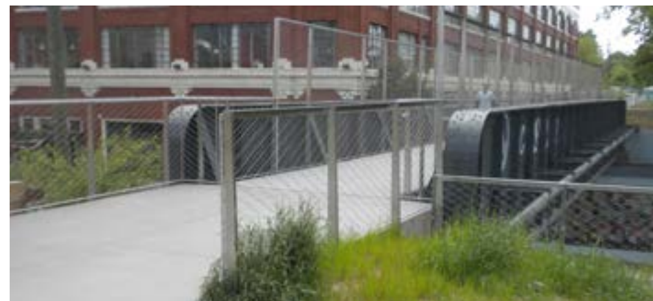
Bridge over Ponce de Leon Ave, a state route, is adapted with state-route compliant missile barrier
