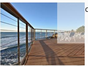
Railing: Cable Railing with 2" steel square tubes and flat steel bar cap
