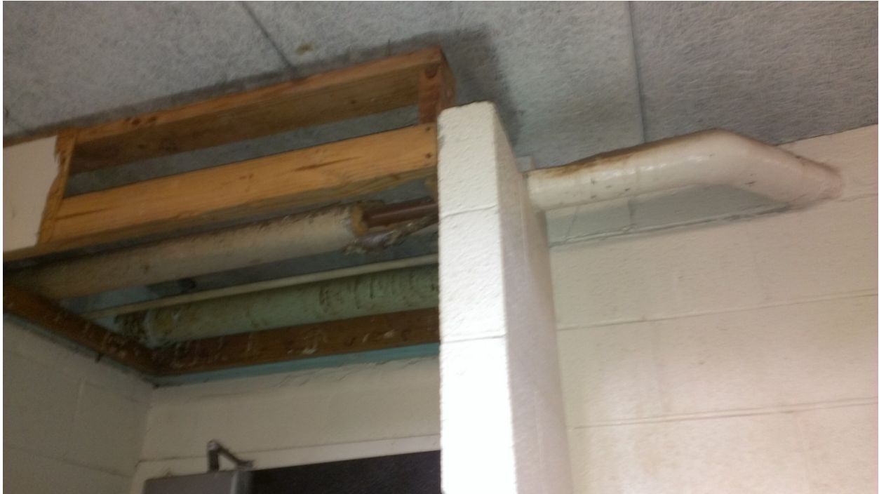
Restroom above the Doorway
