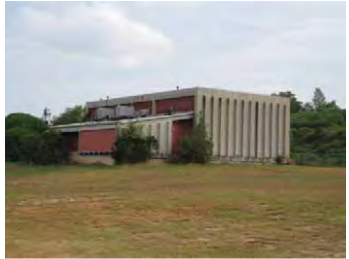
The abandoned recreation center has recently been demolished
