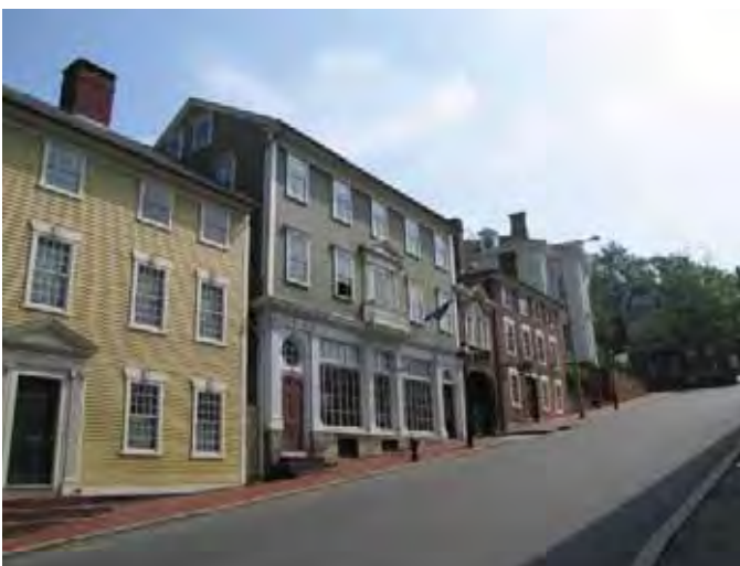
Townhouses and other narrow buildings can easily step up the street within topography
