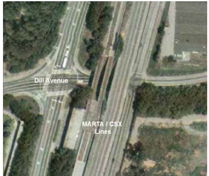
Dill Avenue under MARTA and CSX rail bridges
