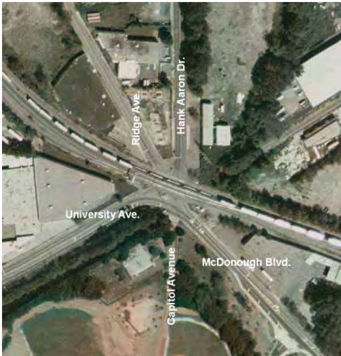
Rail bridge at Hank Aaron Dr./University Ave./McDonough Blvd.
