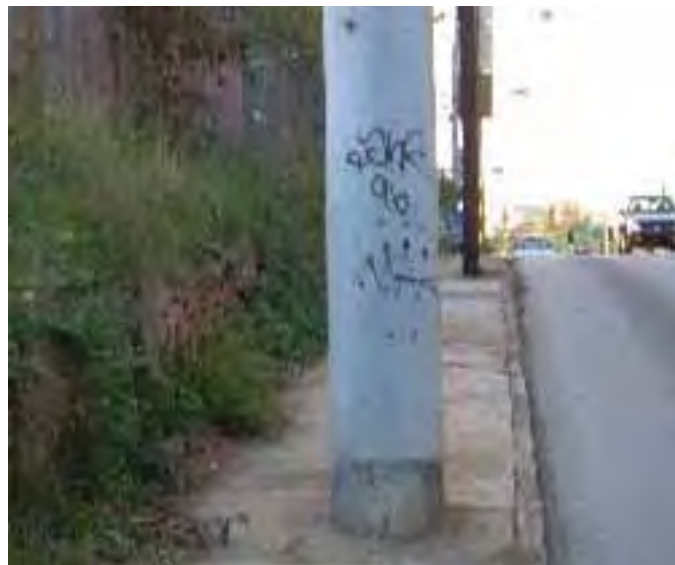
Pole in Sidewalk on Metropolitan Avenue
