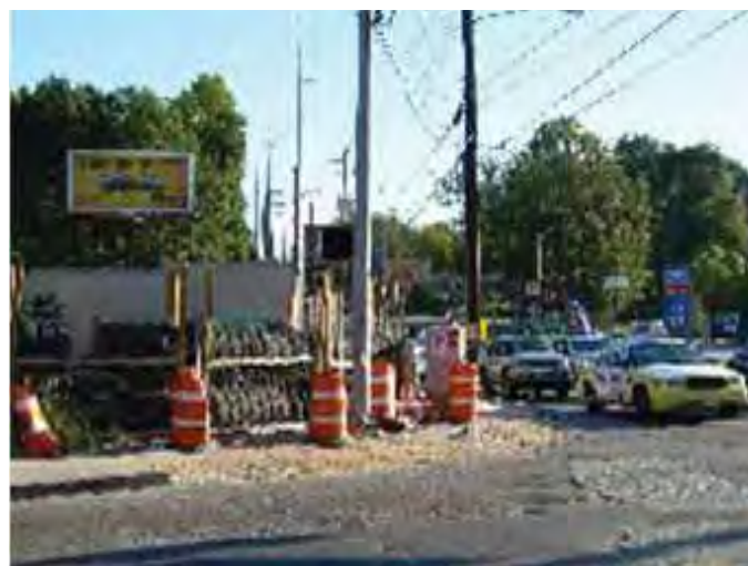
Corner Construction on Metropolitan Avenue
