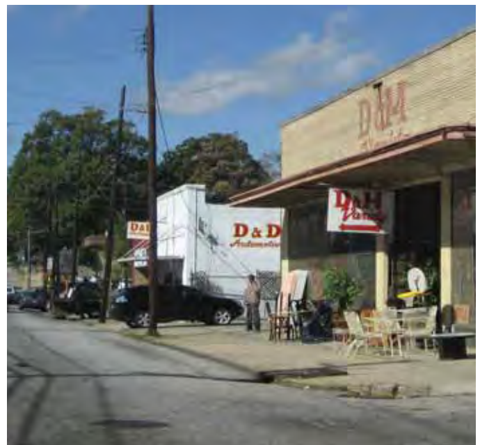
Dill Avenue sidewalks lack wheelchair ramps and are broken in many places
