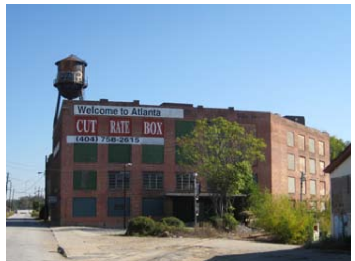
The Cut Rate Box building is a landmark in Subarea 2 and must be preserved
