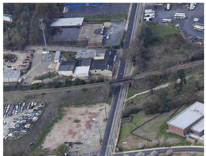
Pryor Road under CSX railroad bridge
