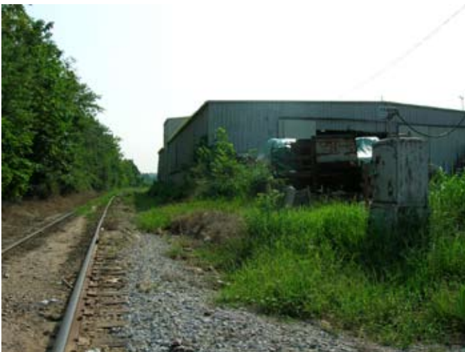
Underutilized industrial land where the BeltLine meets Milton Avenue could become park space
