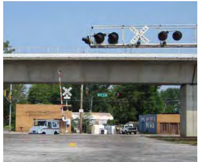
Lee Street/Murphy Street and Whitehall Street
