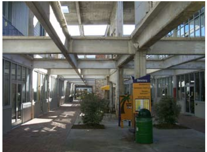
Adaptive reuse of historic buildings in Murphy Triangle could create a unique and memorable space, such as with Atlanta's own StudioPlex in the Old Fourth Ward neighborhood
