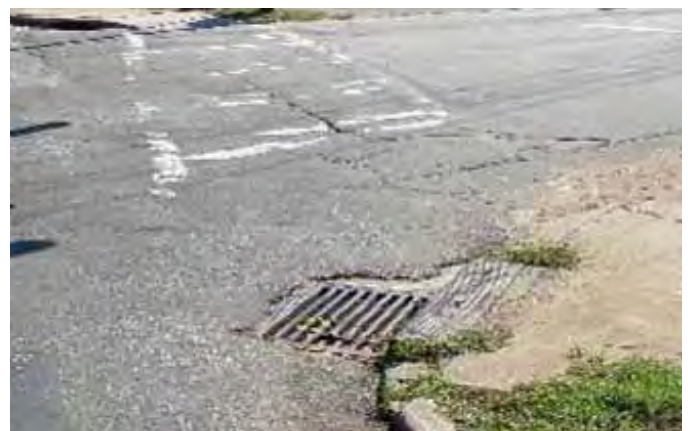
Drainage Grate at McDonough Blvd. and Lakewood Avenue
