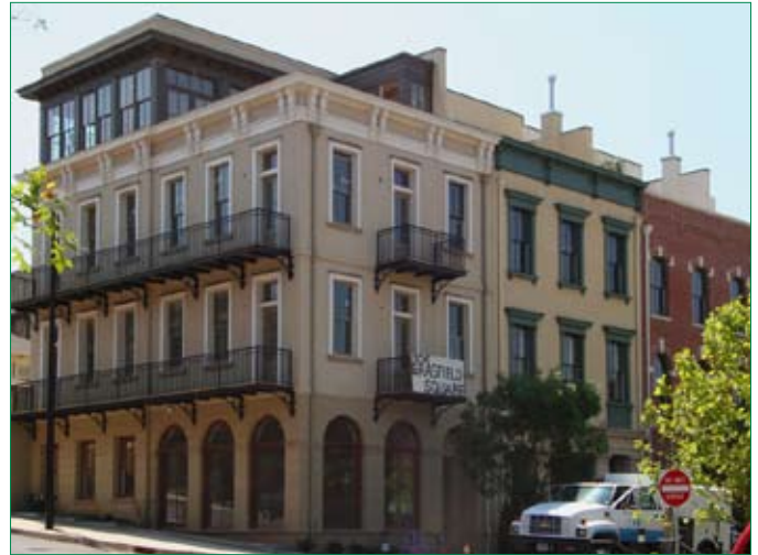
Live/work units in Atlanta's Glenwood Park allow residents to operate businesses out of the first story of their homes. Visitor and employee parking is provided on-street
