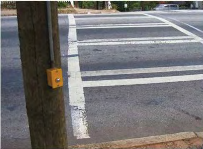
Figure 46 - Pedestrian Button with Inappropriate Placement
