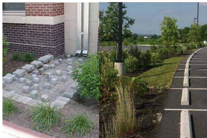
Figure 1 - Example of channeling water runoff into bioretention or rain gardens for water quality and infiltration Courtesy of: Ecos
