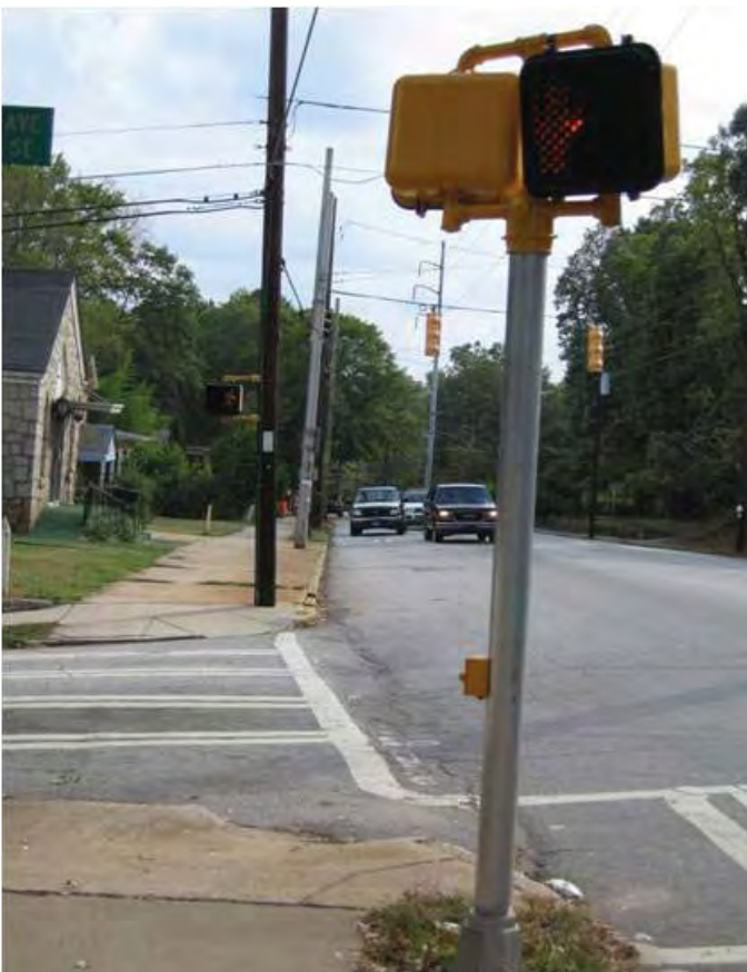
Figure 47 - Disoriented Pedestrian Signal Head
