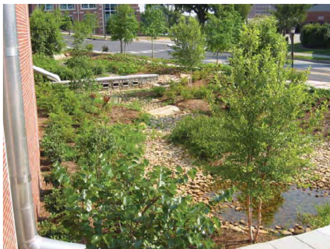
Figure 2 - Example of distributing roof runoff into bioretention areas or rain gardens Courtesy of: Ecos
