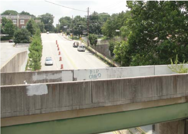
The existing bridge over North Avenue will be adapted for the Atlanta BeltLine trail with safety railings
