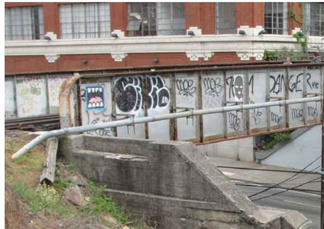
Bridge over Ponce de Leon Ave, a state route, will be adapted with state-route compliant missile barrier
