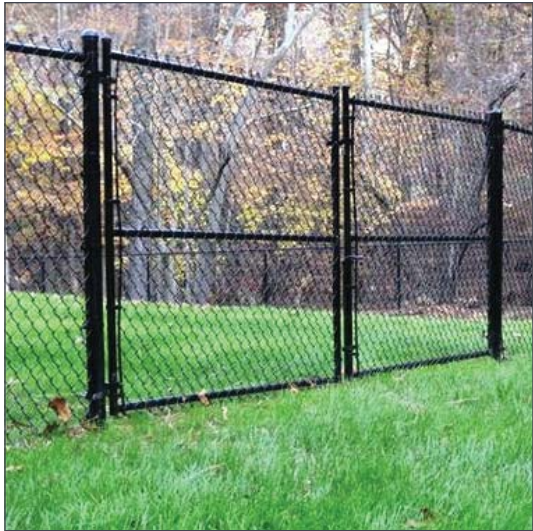
M12 FENCE - TYPE B Chain link fence and screen gates
